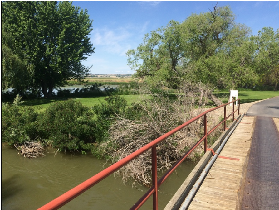
Photograph 8: View west at the west bank of the short span Gamble Island Bridge.
