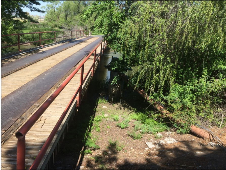
Photograph 7: View west at the vegetation near the east bank of the short span Gamble Island Bridge.
