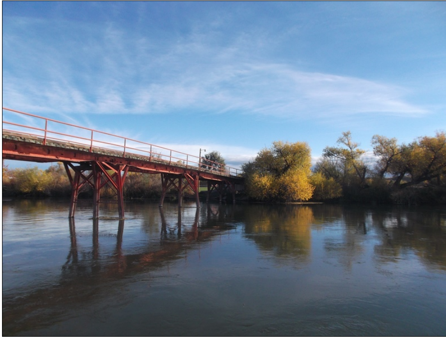
Photograph 3: View from the western bank of the river at the long span Gamble Island Bridge.
