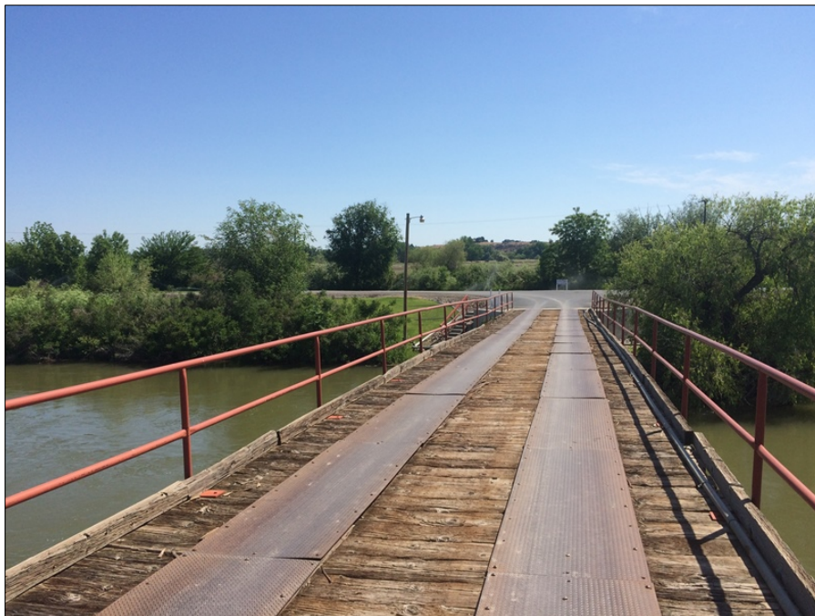
Photograph 6: View east from the center of the long span Gamble Island Bridge.
