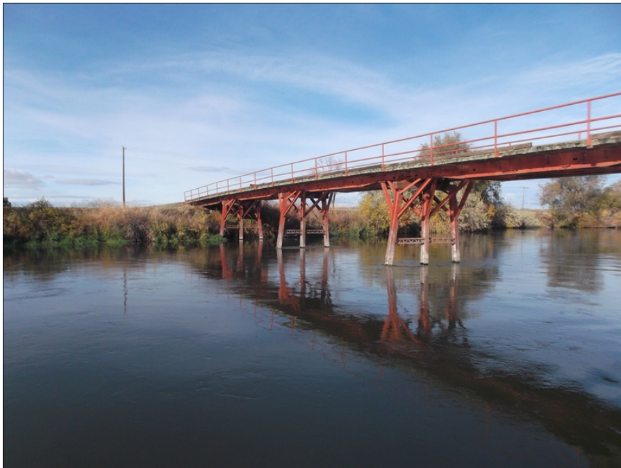
Photograph 4: View from the eastern bank of the river at the long span Gamble Island Bridge.
