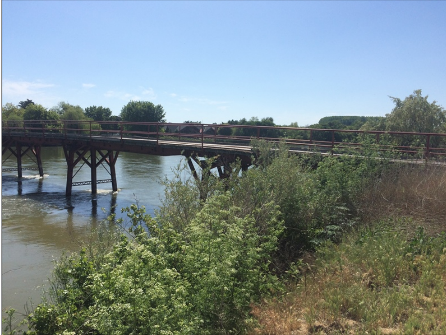
Photograph 5: View from west bank of the Snake River at vegetation near the long span Gamble Island Bridge.
