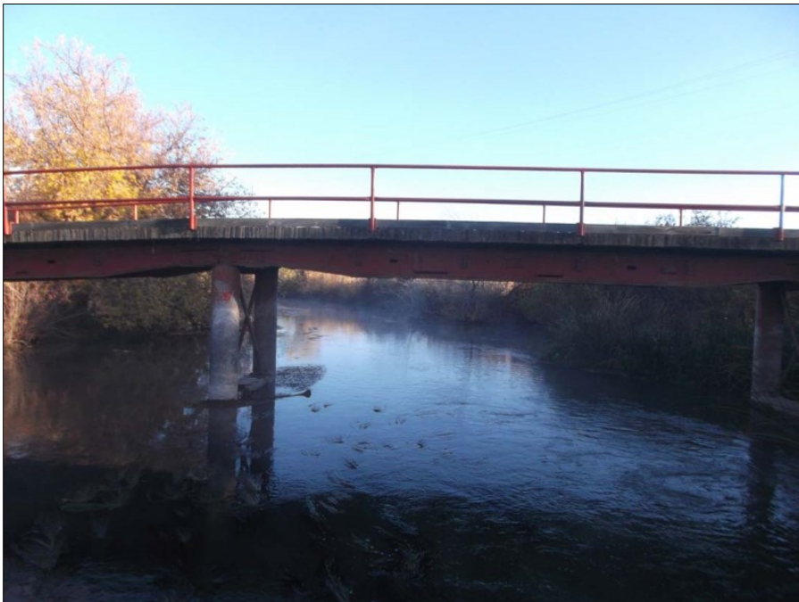
Photograph 2: View north at the short span Gamble Island Bridge.
