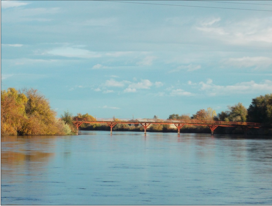
Photograph 1: View north at the long span Gamble Island Bridge.
