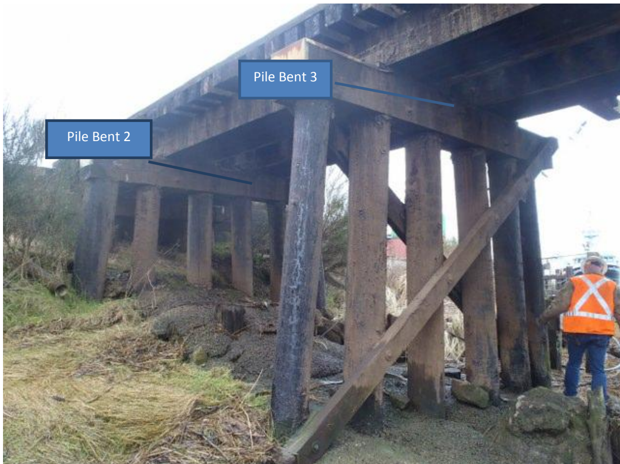
Figure 6. Photo Southwest Showing Wetland Vegetation, Unconsolidated Mud Bottom Under South Approach
