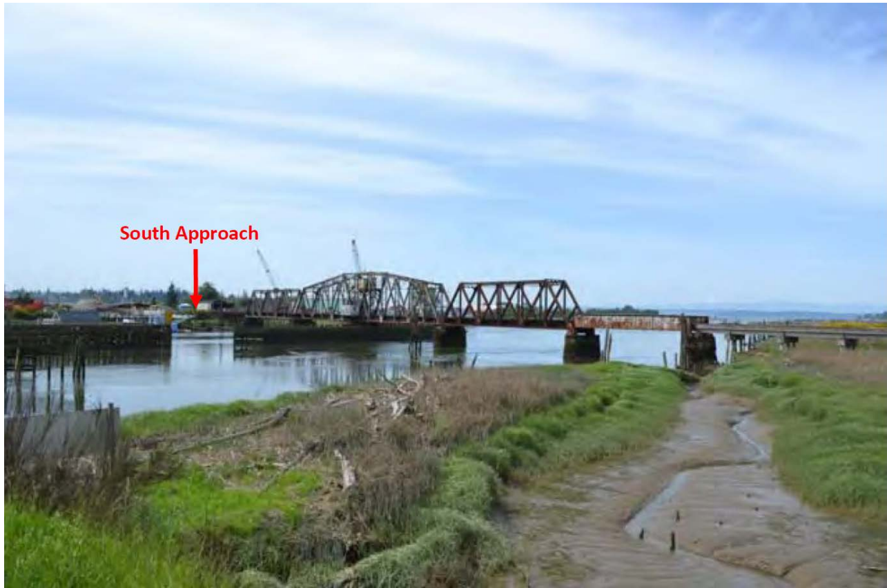
Figure 3. View looking southwest at BNSF Bridge 0050-37.80 near Everett, Washington.
