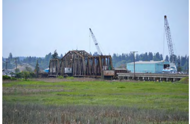
The view is towards the south-southwest from SR 529. The east elevation of the bridge. 2014
