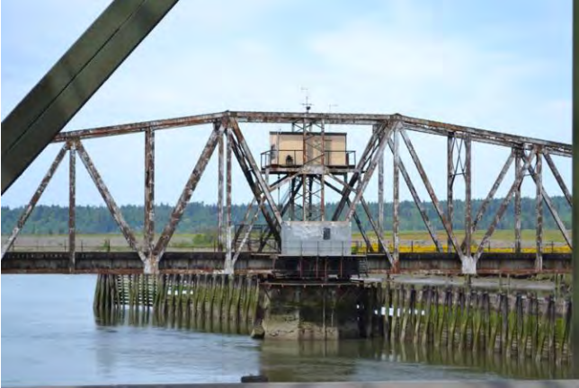
The view is towards the west-northwest from the adjacent southbound SR 529 bridge over Steamboat Slough. Central swing span, control house, and drawrest.
