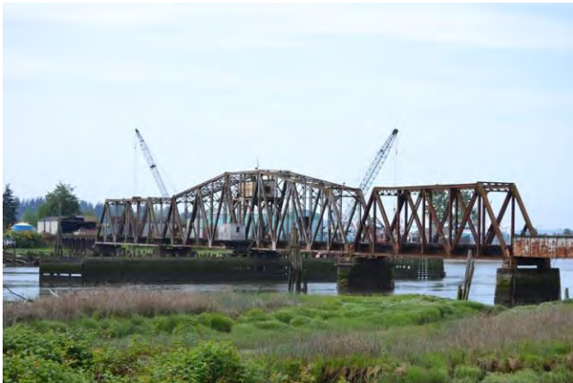
The view is towards the southwest from SR 529. The east elevation of the bridge. 2014
