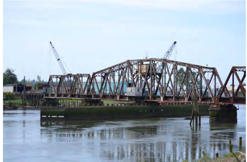
Photo 2. Detail view of the central swing span of BNSF Bridge 0050-37.8. The view is towards the south-southwest.
