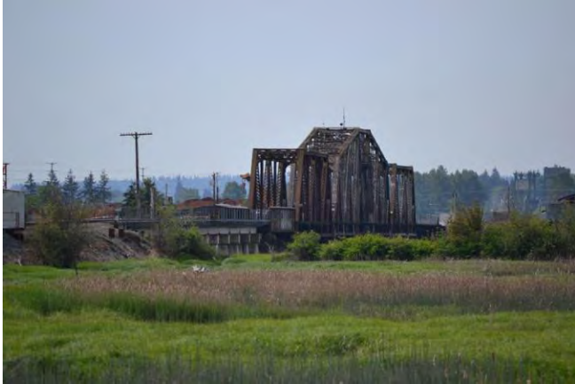
The view is towards the south. The west elevation of the bridge. 2014
