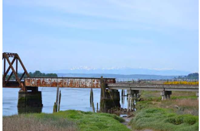
The view is towards the west-southwest from SR 529. The through plate girder that connects the replacement north approach (right) to the northernmost steel truss (left).
