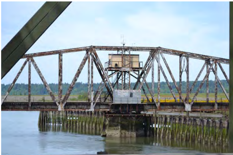
Photo 3. Detail view of the central swing span and control house looking west-northwest from the adjacent SR 529 southbound bridge over Steamboat Slough.
