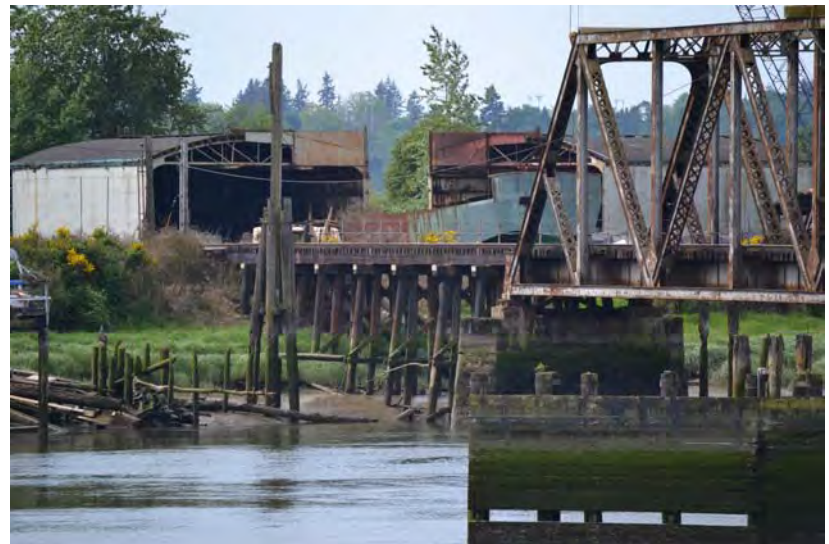
Photo 4. The south approach of the bridge, which currently consists of an 8-span timber pile trestle, will be replaced with a 4-span pre-stressed concrete double cell box girder. The view is towards the south-southwest.
