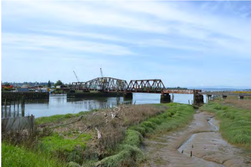
Photo 1. Overview of BNSF Bridge 0050-37.8 at Steamboat Slough. The view is towards the southwest from southbound SR 529.
