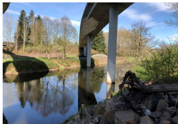
Northbound I-405 to eastbound SR 522 ramp with two piers proposed for removal in the Sammamish River.
